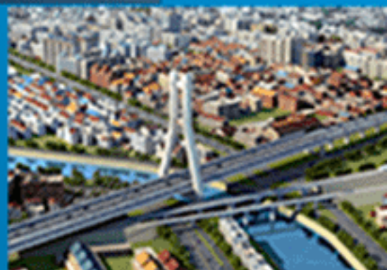
Fujian Longyan Avenue viaduct
