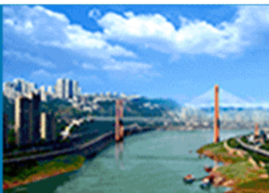
Jialingjiang bridge in Hongyan village, Chongqing
