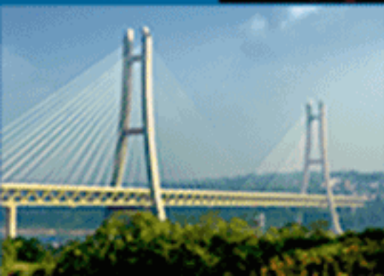
Chongqing Dingshan Yangtze River Bridge
