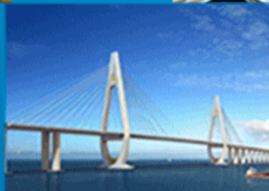
DSSG02 bid section of Ningbo Zhoushan port main channel
